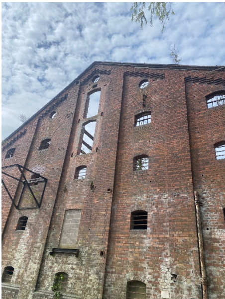
Gable eastern end:
